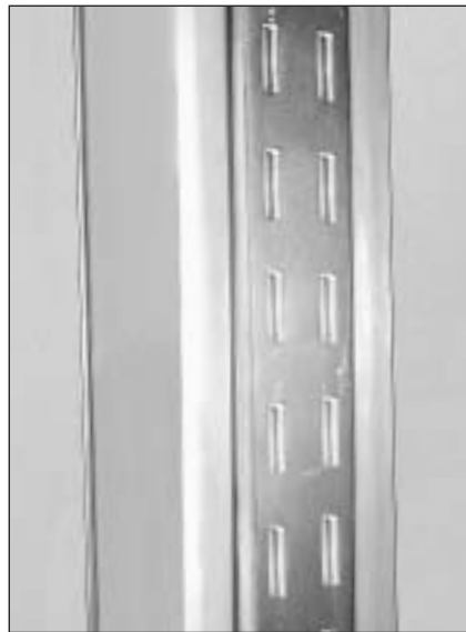
Rear view of outrigger shows double slotted steel standards mounted to aluminum post.
